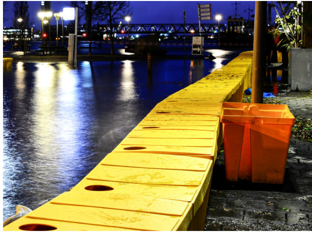
Figure 1: Temporary flood barriers. Photo credit: Boxbarrier b.v.
